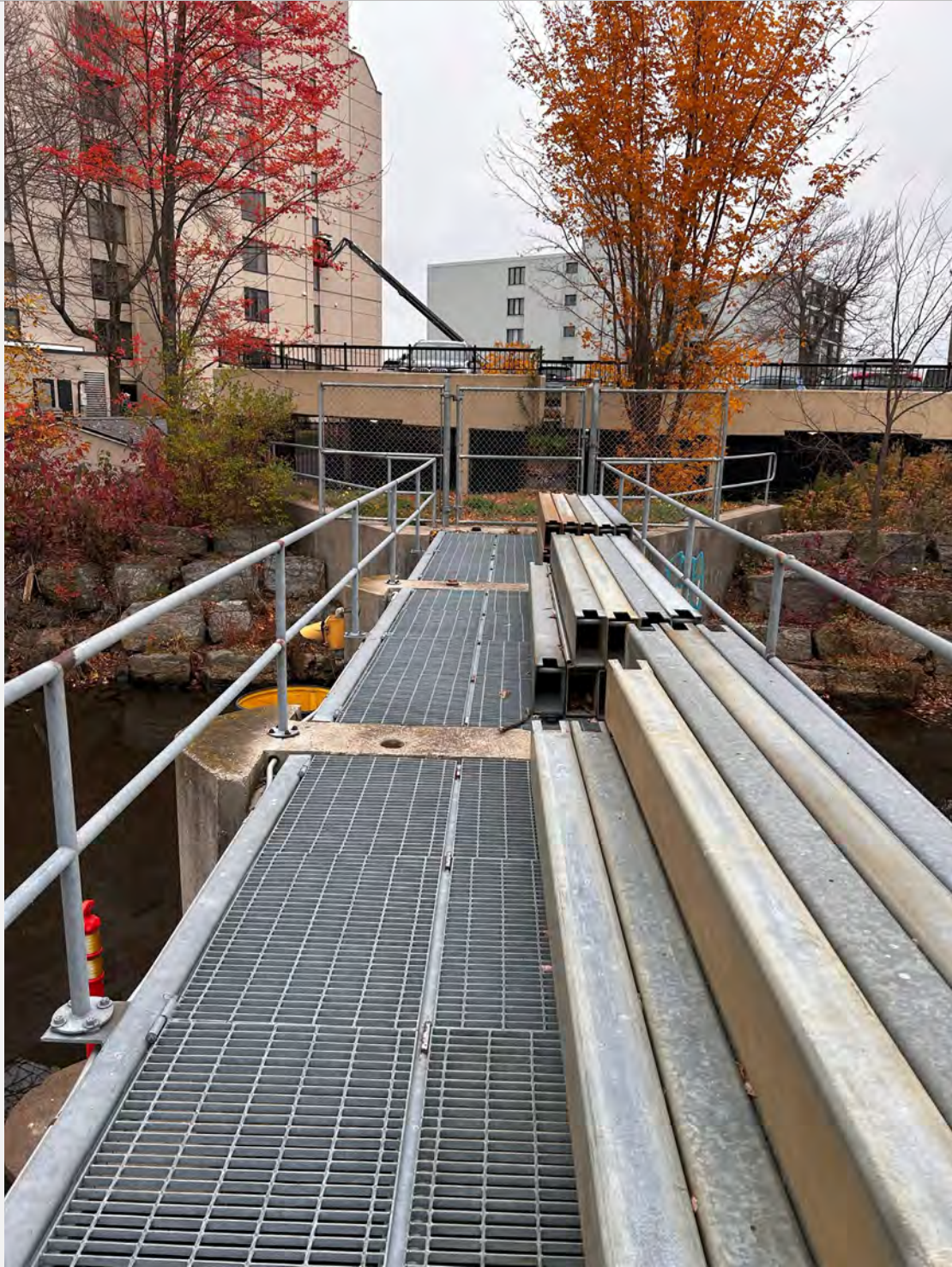
Galvanized Metal Deck, Supports and Barrier Railings
